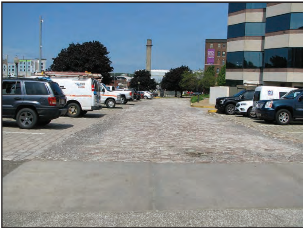
Dobbins Lane looking northeast from Peach Street.
