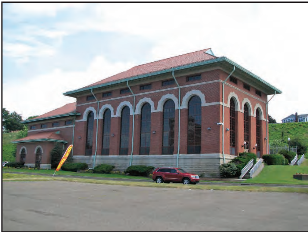
Erie Waterworks, Pump House (1913/2001).
