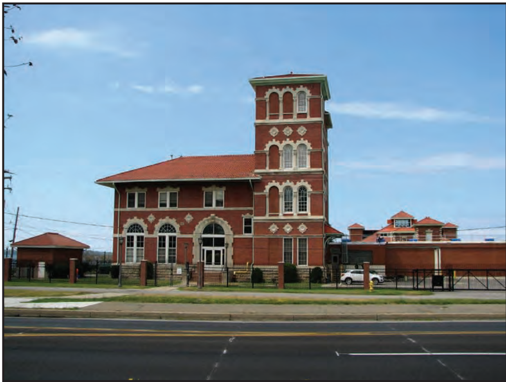
Erie Waterworks, Filtration Building (1913).
